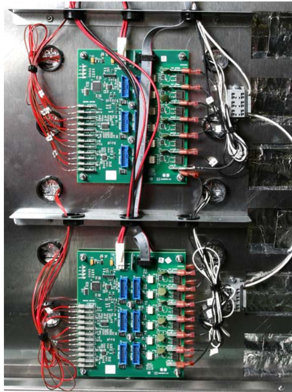
Fig. 7: Distribution board shown with display cables removed.
