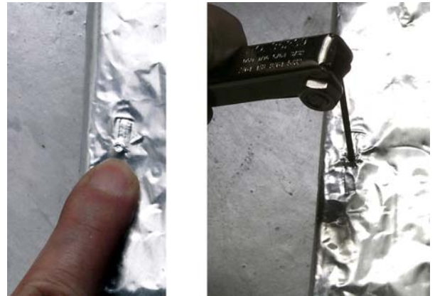
Fig. 11, 12: Find the set screws under the foil insulation and push through with an allen wrench.
