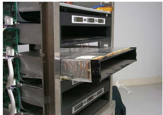
Fig. 17. Slide malfunctioning slot from cabinet.
